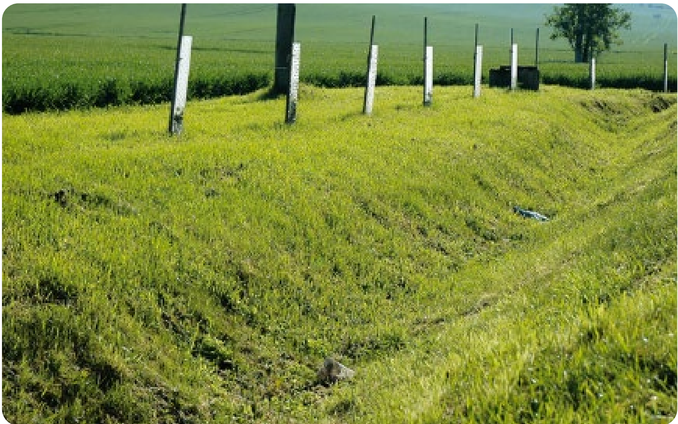
Grassed retention ditch as designed in the Czech Republic (Dzuráková et al., 2017)
